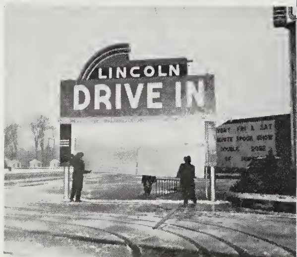
Display and name signs should also be boarded up during the winter shut-down period. However, the bulbs should be left in or sockets will corrode.
